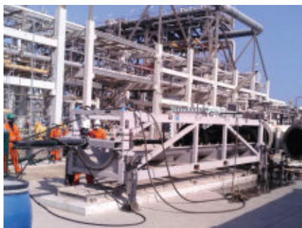
STATS Group working on a Remote Tecno Plug project in Qatar.
