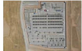
Drone overview of the project.
