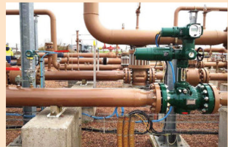
The unit allows for remote pressure control
