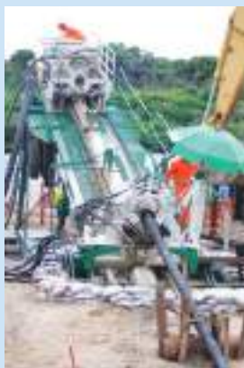
Horizontal drill rig at 16 degrees.
